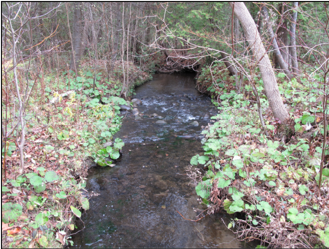
Photo 7: Reach 3 - There is some active erosion within the channel.
