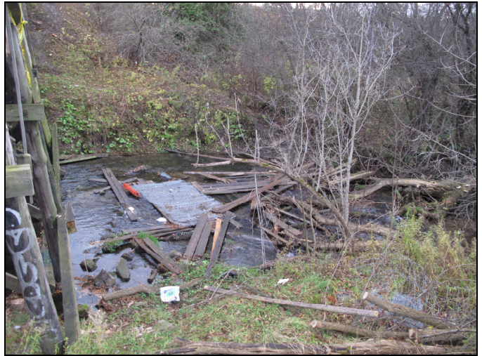
Photo 16: Reach 19 – Refer to Figure ERSN 1 for location of shot. Several debris in channel at the bridge area.
