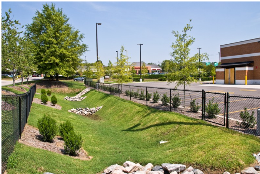
Grassed Drainage Swale w/ Rock Check Dams
