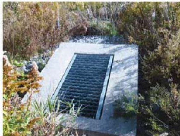
Outlet structure, DICB
