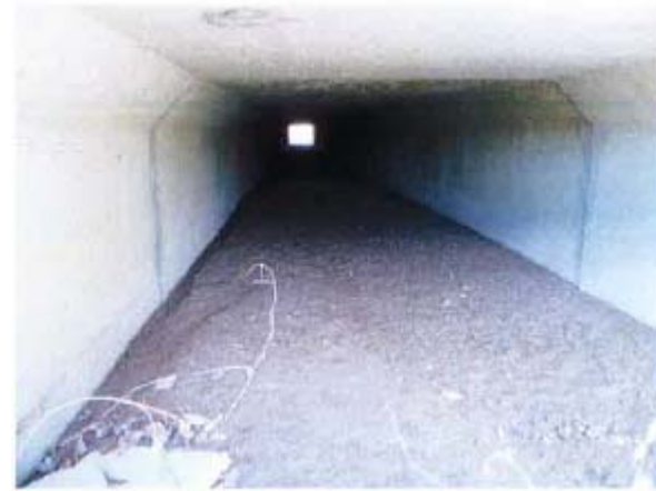
Central headwall culvert
