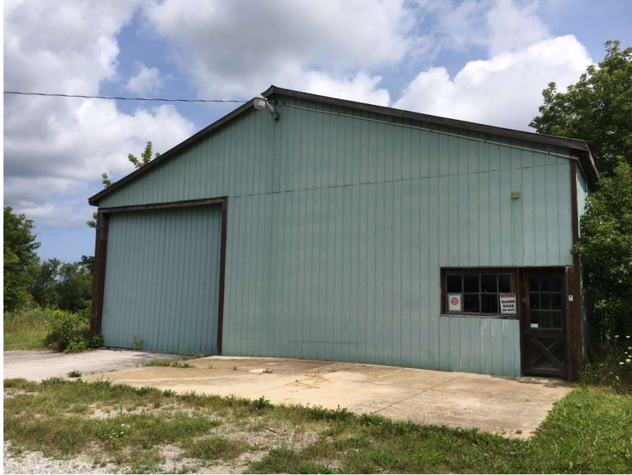
Photo 5: Front of metal clad maintenance building on east side of driveway.
