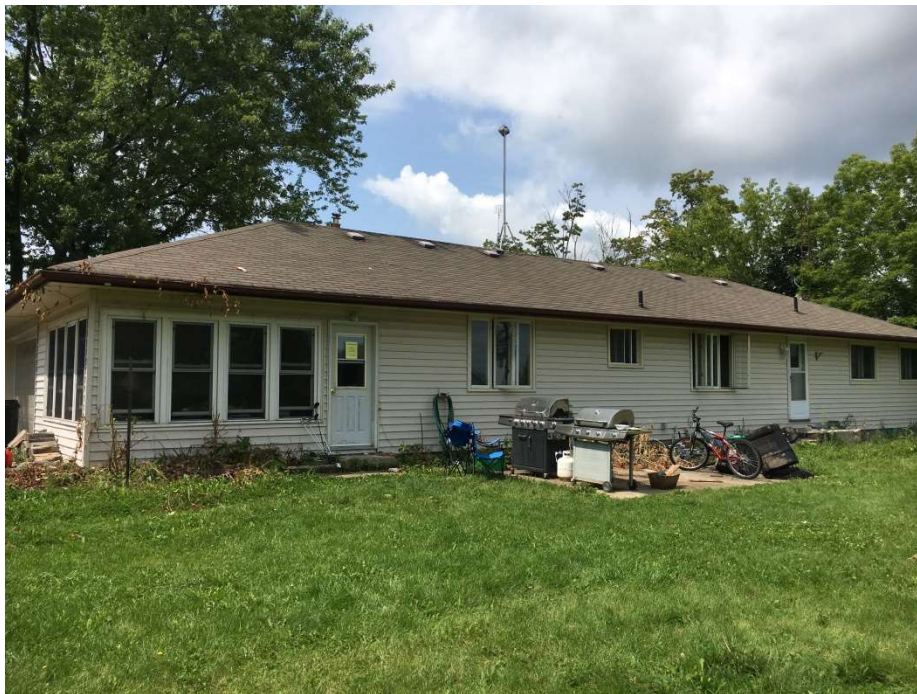
Photo 20: East side of residential dwelling near driveway exit/entrance at Dafoe Street.
