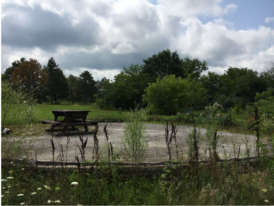
Photo 13: Concrete foundation of former silo on west side of driveway.
