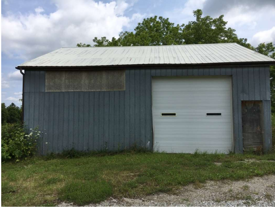
Photo 3: Looking east at the metal clad storage building on the east side of the driveway.
