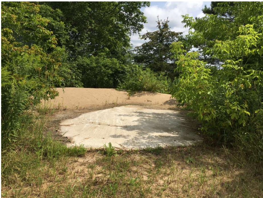
Photo 14: Concrete foundation of former silo, southwest of the maintenance building.
