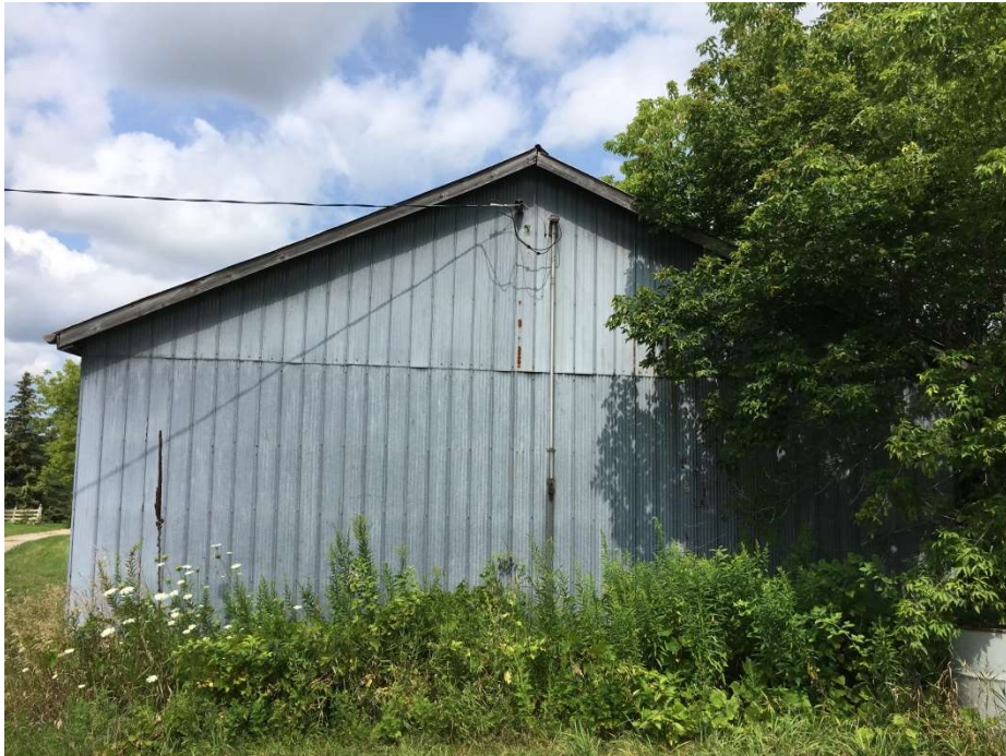
Photo 4: South side of storage building.
