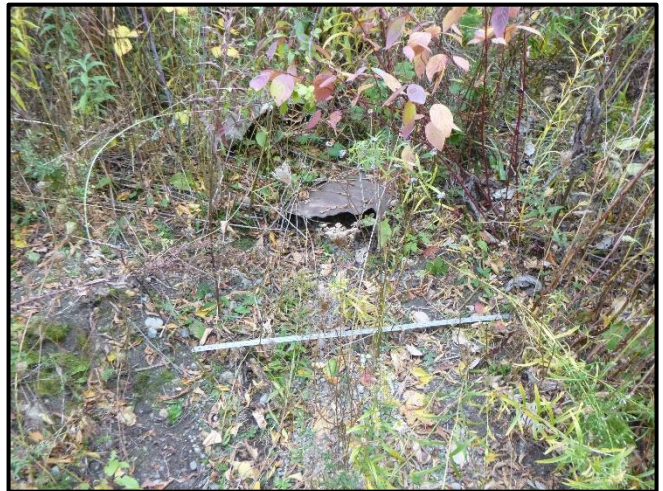
Photograph 4. Reach UBTA-1 Upstream view of existing culvert.
